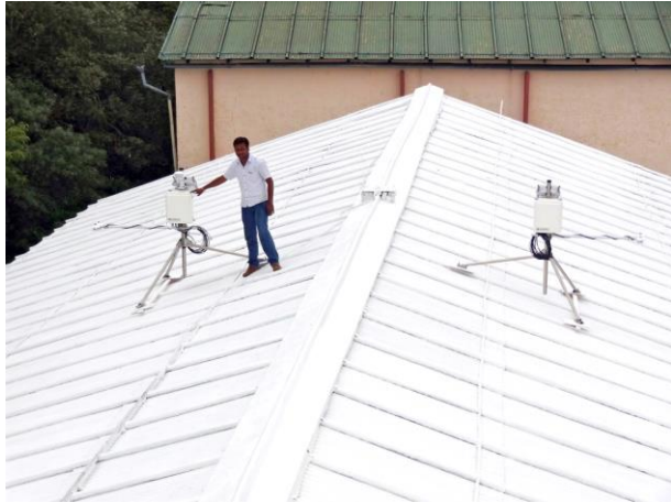
Cool roofs can reject 90% of the heat energy that lands on them, reducing the need for ACs.
