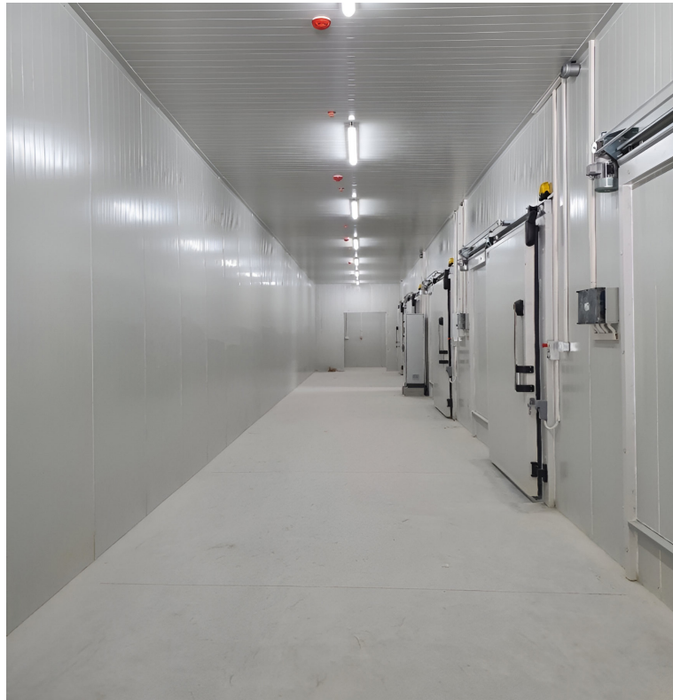
Figure 14: Photo of an ante-room
