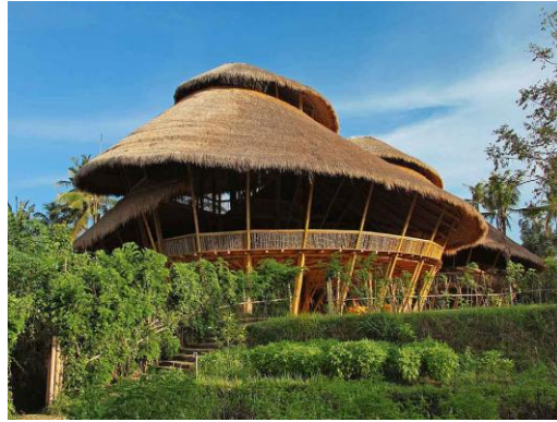
Figure 11. Kul-Kul Farm at Green School Bali Source: [101]
