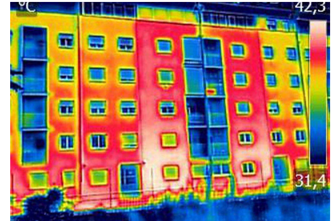
Overheating in buildings
