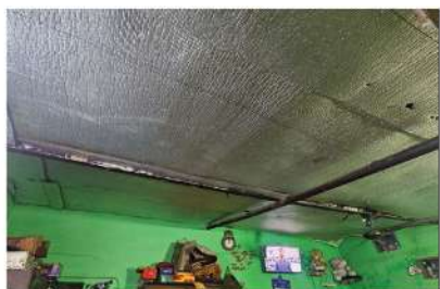
XLPE (Cross linked Polyethylene) Foam Sheets fixed to the ceilings
