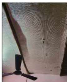
XLPE (Cross linked Polyethylene) Foam Sheets fixed to the ceilings
