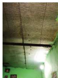
XLPE (Cross linked Polyethylene) Foam Sheets fixed to the ceilings
