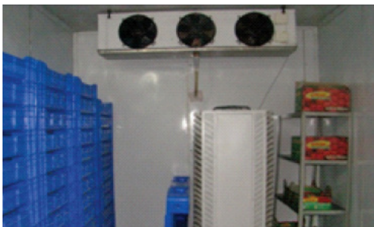
Figure 8: Litchi Cold Storage
