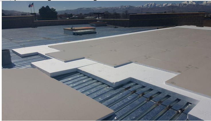
Figure 34 XPS insulation application procedure 19
