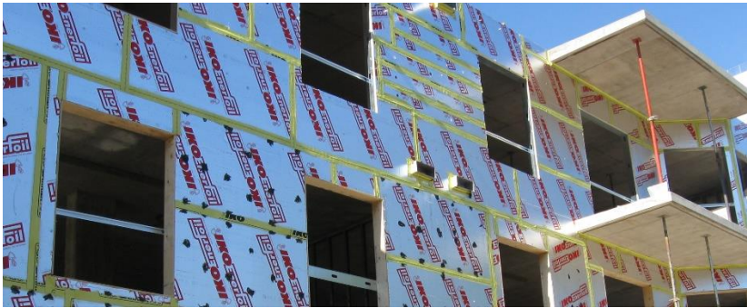
Figure 25 Polyisocyanurate foam board insulation application procedure 13
