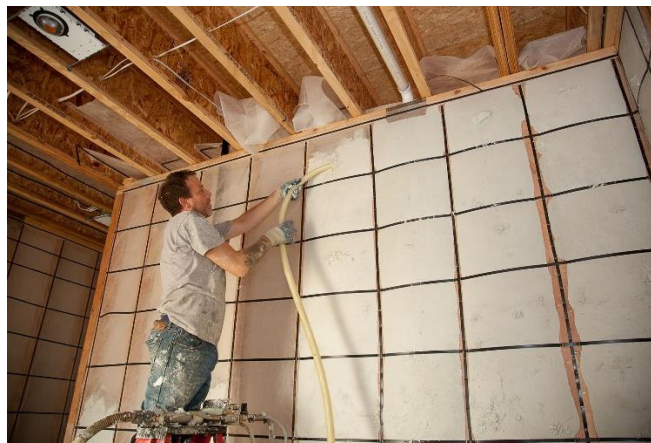
Figure 27 Cementitious foam insulation application procedure 15
