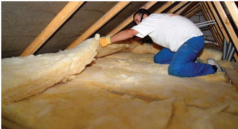
Figure 35 Glass wool insulation application procedure 20
