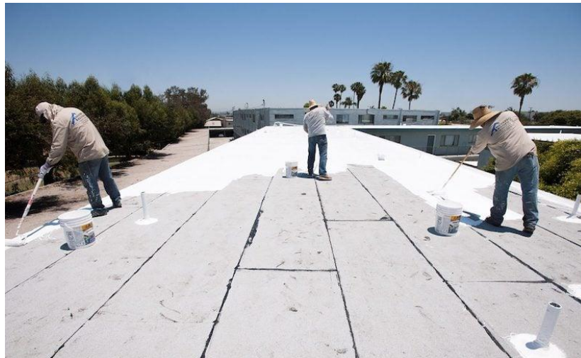
Figure 30 Reflective/ cool paint application procedure 17
