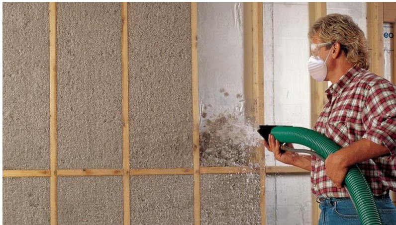
Figure 23 Cellulose insulation application process 11
