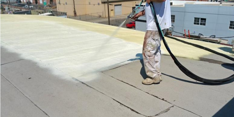
Figure 33 PUF spray insulation application procedure 18
