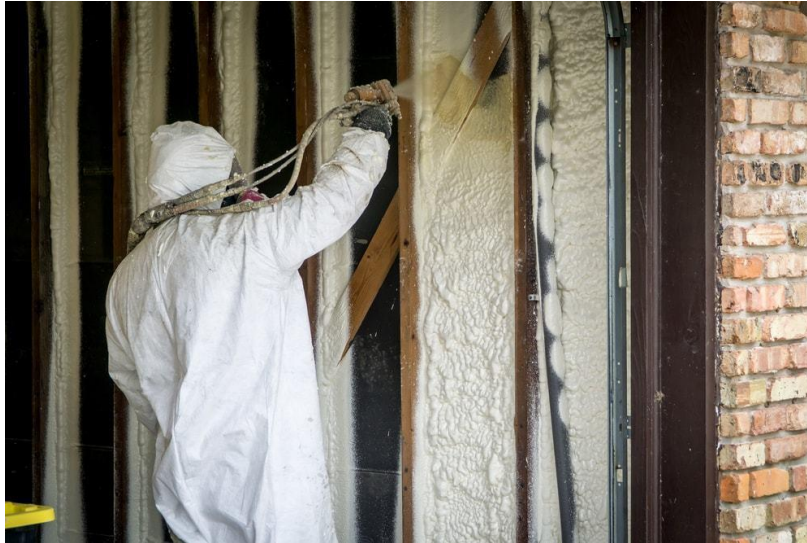
Figure 26 Polyurethane insulation application procedure 14
