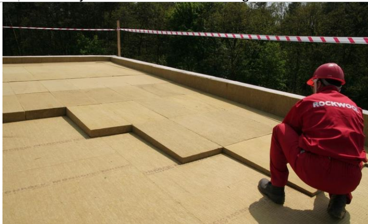
Figure 36 Rock wool insulation application procedure 21
