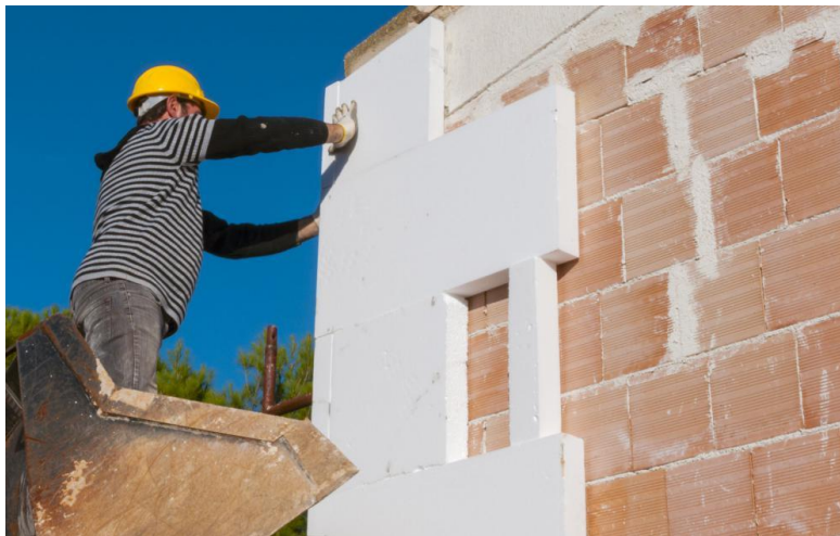
Figure 24 Polystyrene insulation application procedure 12
