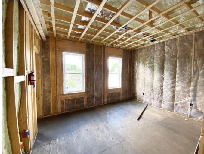
Figure 22 Mineral wool insulation application procedure 10
