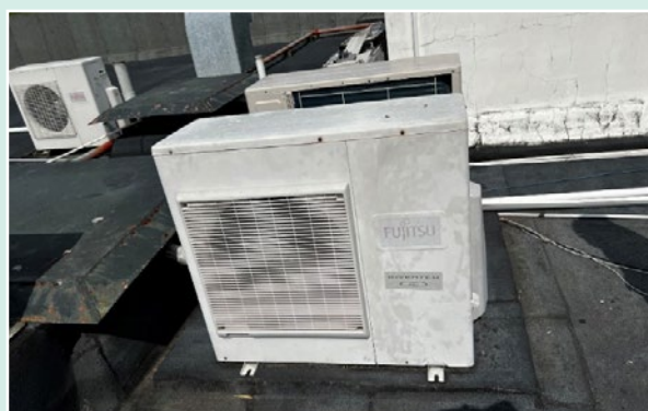
Installed condensing unit (On-site)
